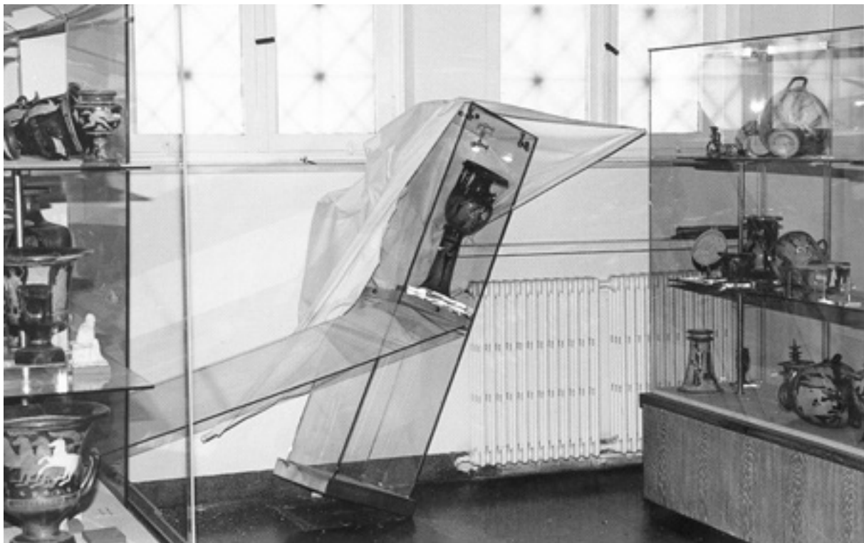
Fig. 3. Failures caused by overturning at the National Museum of Athens during the 1999 Athens (Parnitha) earthquake (Spyrakos et al. , 2008).
